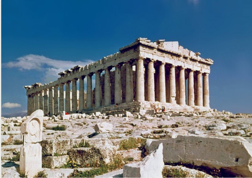
The Parthenon, Athens, 447-438 BC, a peripteral octastyle Doric temple on a curved stylobate and multi-drum shafts with entasis on top of which is an echinus and abacus supporting an entablature consisting of triglyphs (with mutules and guttae) and metopes, below a pediment whose tympanum contains sculptures
