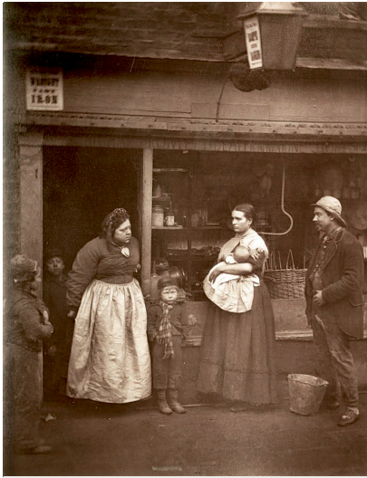
Street Floods in Lambeth
