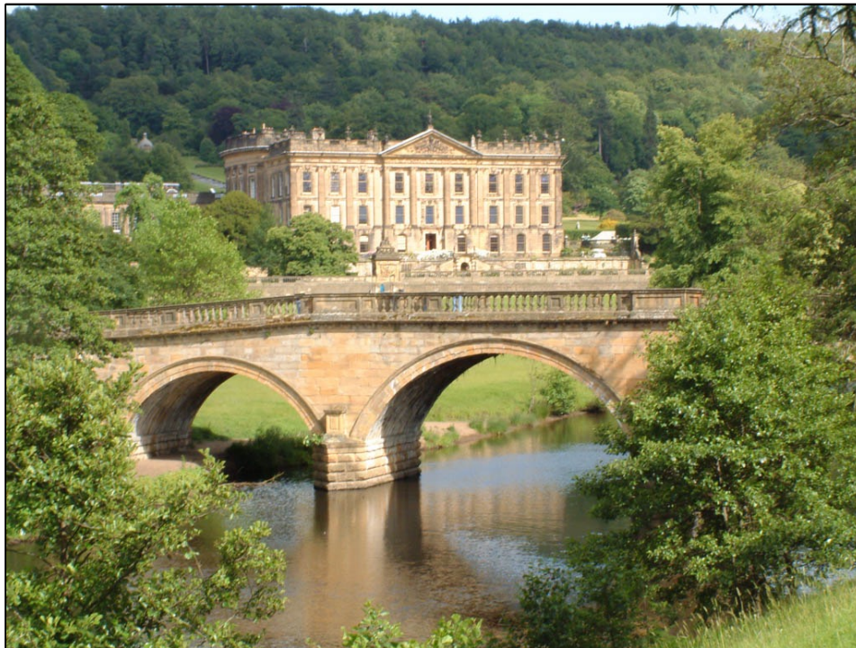
William Talman (1650-1719), Thomas Archer (1668-1743), Jeffry Wyattville, Joseph Paxton, James Paine Chatsworth House, south façade 1696 Architecture Chatsworth House, Derbyshire
