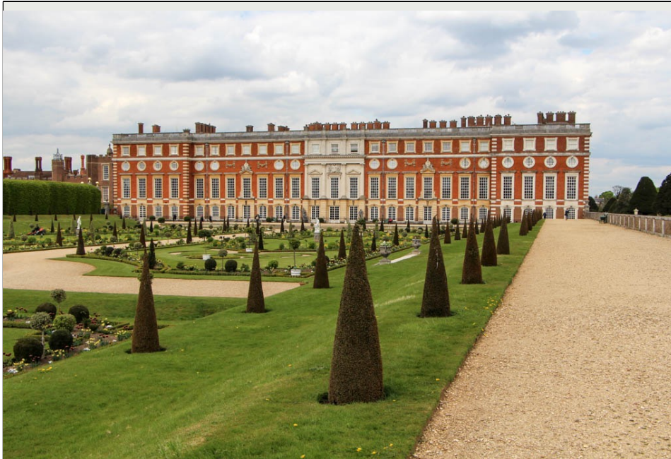
Christopher Wren (1632-1723) and William Talman (1650-1719) Hampton Court, south facade 1689-1702 Hampton Court Palace, East Molesey, Surrey
